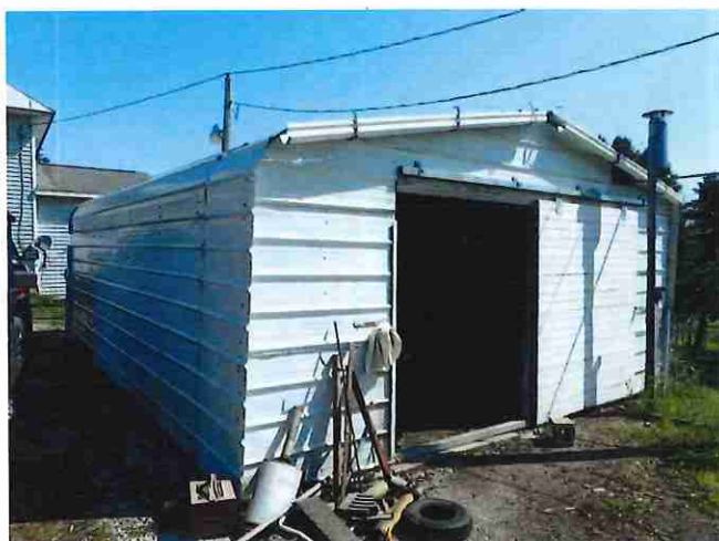
Wood Burner Shed
